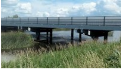
Gudenå piledeck Requalification, 1993
