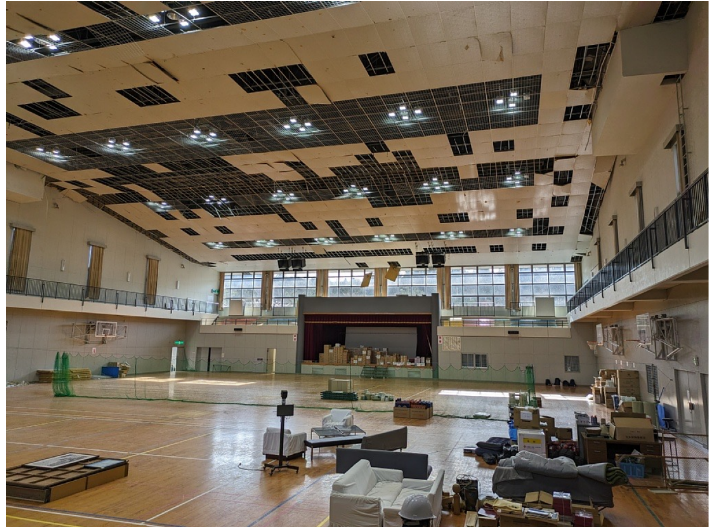
Suspended Ceilings in a Public Gymnasium
